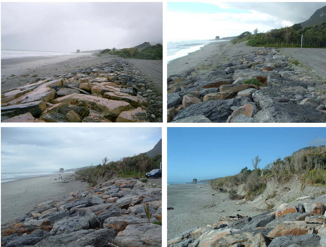
Figure 1: Beach and dune changes at the northern end of the rock revetment at Punakaiki over the last year: Top left: November 2005, Top right: May 2006, Bottom left: November 2006, Bottom right: December 2006.
