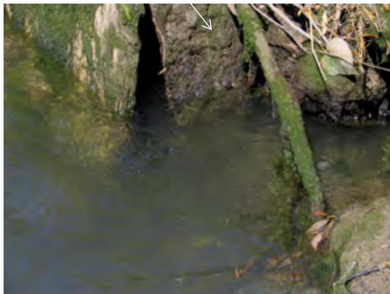
Figure 3. Motueka tide gate remains open even at half tide height, allowing about four to six hours on every tide cycle for whitebait to negotiate the culvert.
