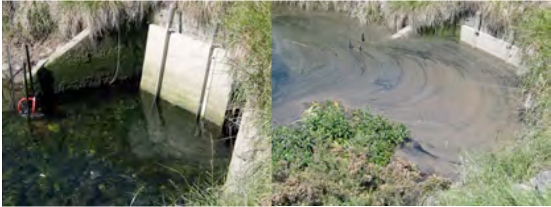
Figure 6. Pearl Creek tide gate open at low tide (left) and closed at high tide (right). DIDSON is mounted between three waratahs at left of frames. On the tide monitored, water eventually covered the top of the waratahs and the tide gate.
