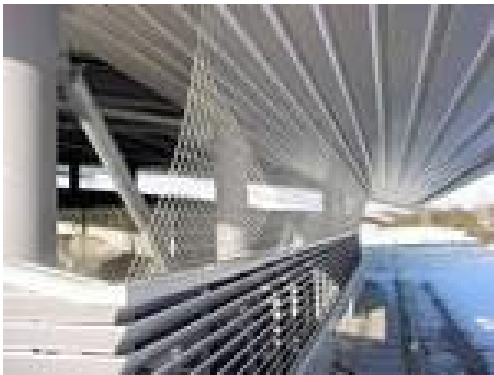
Fig. 5 Netting (photo sourced from http://www.pigeoncontrolresourcecentre.org/html/reviews/wire-mesh-exclude-nuisance-pigeons.html , accessed 8 July 2009).
