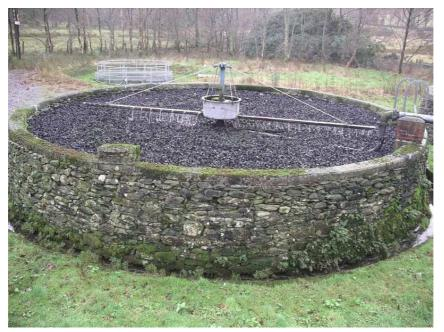
Figure 1 Trickling filter bed using plastic media for secondary sewage treatment
