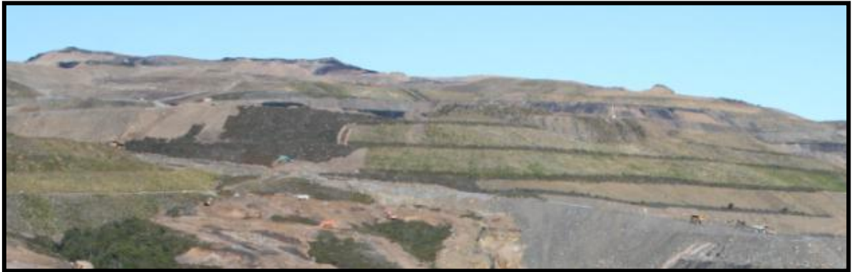
Figure 21 Typical engineered overburden landforms for long-term stability. Many benches have a line of VDT (dark green vegetation) at the top and bottom of each batter to assist erosion control (2012).
