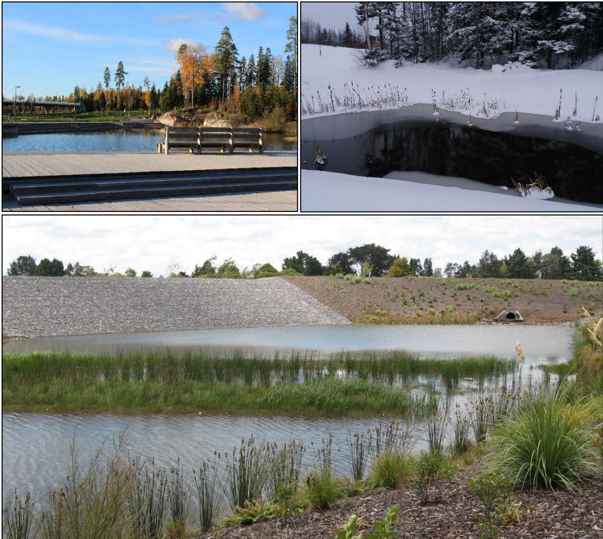
Figure 2-3: Wet retention ponds in Tampere, Finland (top) (pictures from Eisenberg and Polcher (2019) and Auckland (lower). (picture from Dr Annette Semadeni-Davies).
