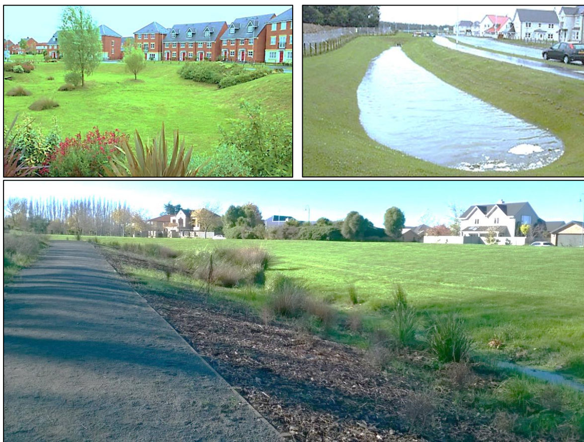
Figure 2-4: Dry detention pond and infiltration basin (top left) (Source: susdrain.org) and vegetated swale (top right) (sudswales.com) in United Kingdom; and vegetated swale in Christchurch New Zealand (Source: niwa.co.nz).
