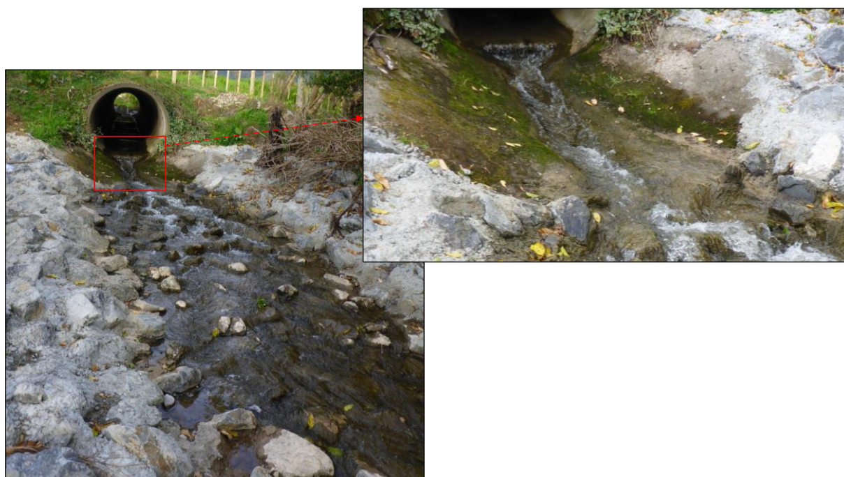
Figure 6-1: Remediated culvert on Kara Stream, Upper Kingston Road. Inset shows the unmodified culvert apron.
