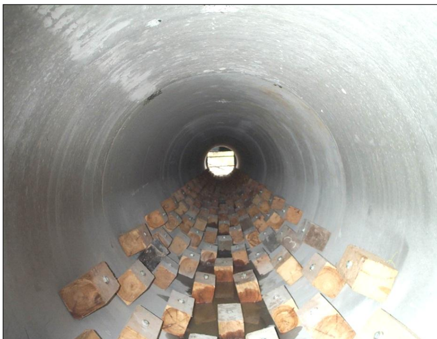
Figure 6-16: Wooden spoiler baffles (0.25 m length, 0.12 m width and 0.12 m height) installed in a 1.3 m diameter culvert. Spoiler baffles are attached to the concrete with stainless steel bolts.
