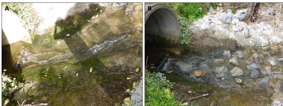
Figure 6-3: Culvert apron at Upper Kingston Road. A, unmodified. B, modified using boulders as baffling elements.
