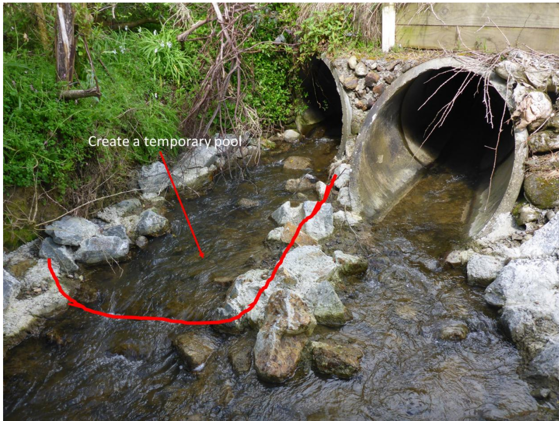
Figure 5-3: Recommended area to create a temporary pool to facilitate testing inanga passage through the baffled culvert in Kara Stream at Lower Kingston Road. Utilise sandbags and/or rocks to form the pool boundary.
