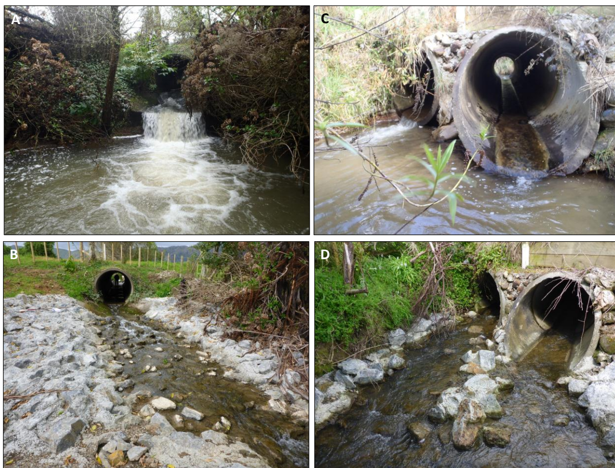
Figure 2-1: Rock-ramps created to enhance passage of both swimming and climbing fish species in Kara Stream, Manawatu. A, Upper Kingston Road culvert before remediation. B, Upper Kingston Road culvert after remediation. C, Lower Kingston Road double culvert before remediation. D, Lower Kingston Road double culvert after remediation.
