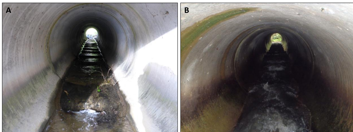
Figure 6-2: Culvert under Upper Kingston Road. A, at low flow. B, at high flow.
