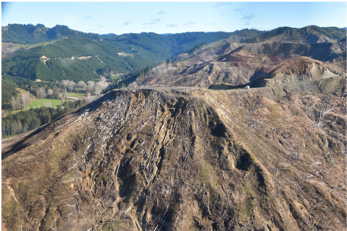
Figure 4.8 Soil slides and debris flows with source areas in fill used to construct a landing in the Mangatoitoti Stream, Mangaheia catchment near Five Bridges (Uawa Forest) (D. Townsend, GNS Science; 11 July 2018; D85_8035).
