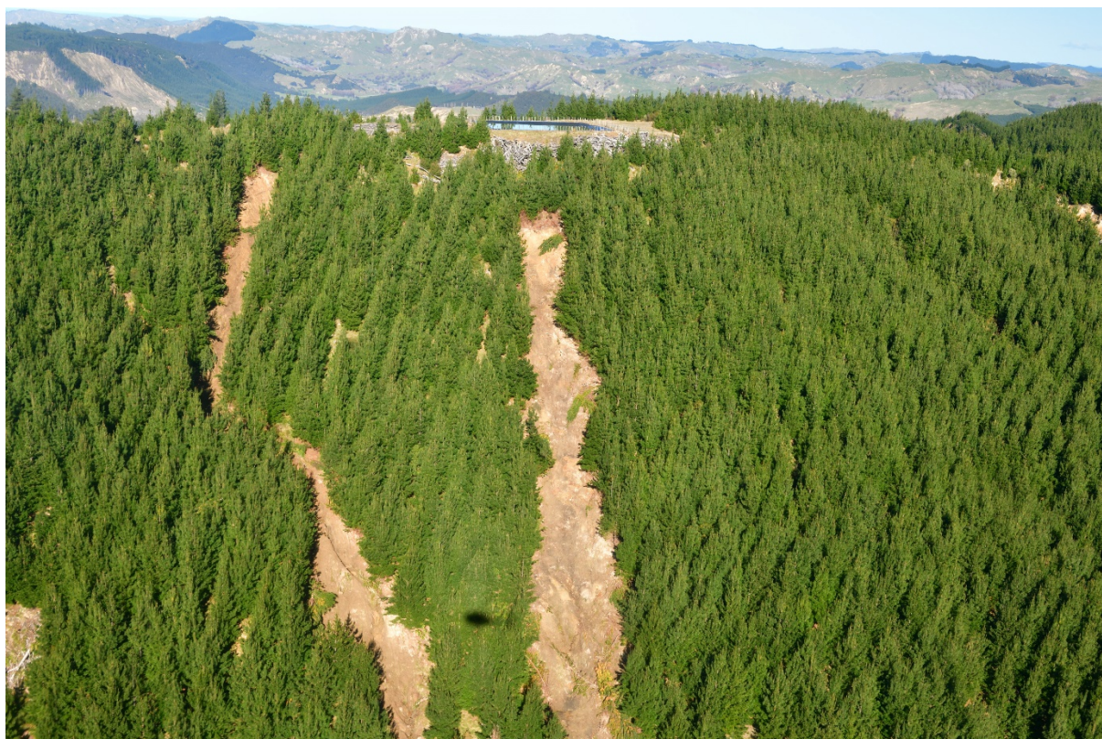
Figure 4.5 Debris flows initiated in established pine plantations in the headwaters of the Mangatokerau River (Te Mauranga Forest). The right-hand debris flow may have initiated in fill associated with the water reservoir visible on the ridge crest (D. Townsend, GNS Science; 11 July 2018; D85_7879).
