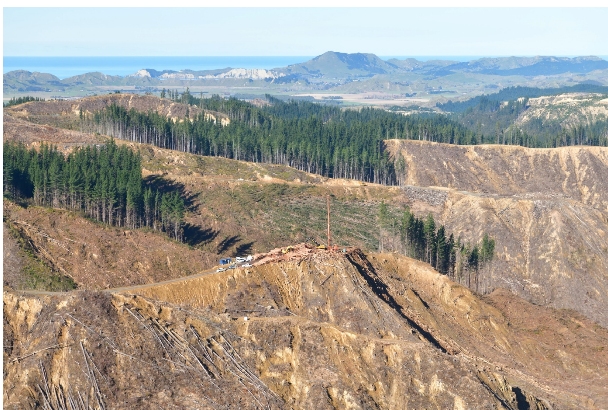
Figure 4.6 Skid haul operation in a newly harvested area in the head of Tapuae Stream, Paroa Forest, Uawa catchment. Shallow soil slides have initiated in the fill slopes constructed for landings and roads built to facilitate harvesting operations (D. Townsend, GNS Science; 11 July 2018; D85_7887).
