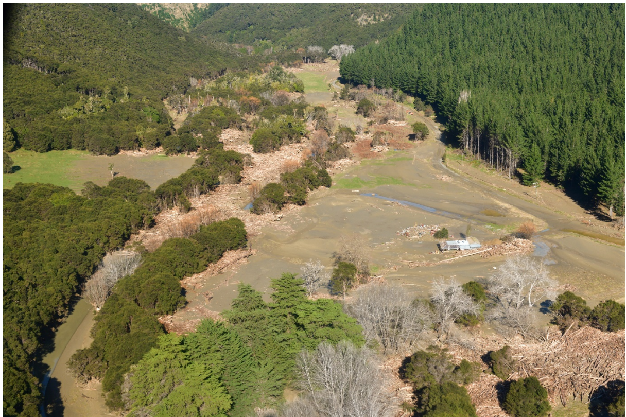
Figure 4.16 Woody debris deposited on the floodplain of the Mangatokerau River upstream of the Paroa Road Bridge showing Mangatokerau Road where 3 people were rescued during the Queen's Birthday Storm (D. Townsend, GNS Science; 11 July 2018; D85_7913).
