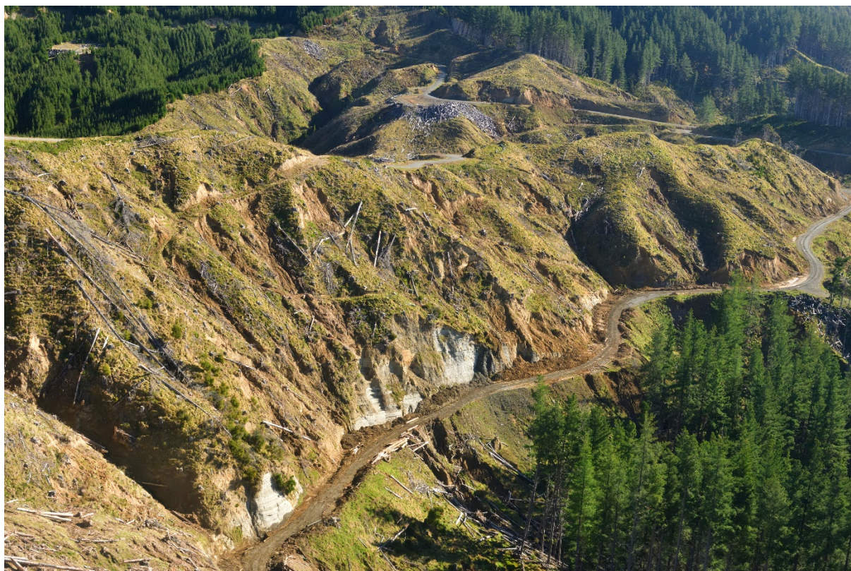
Figure 4.10 Soil and rock falls, soil and rock slides, and soil flows originating on or above cut slopes above Tirohanga forestry road between Kaimonona and Te Kokokakahi Streams in the headwaters of Mangatokerau River (D. Townsend, GNS Science; 11 July 2018; D85_7872).
