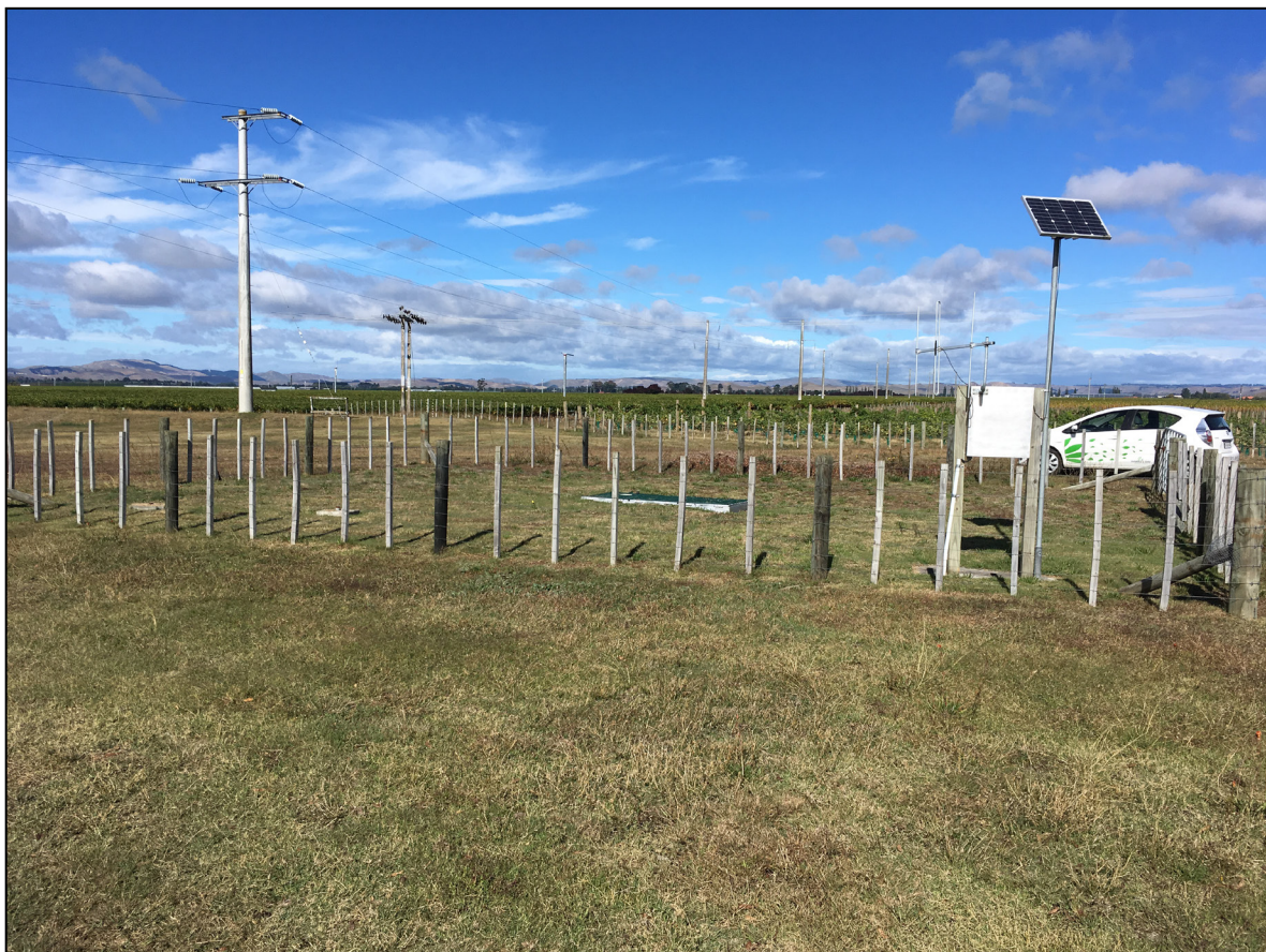
Figure A4.2 Substation lysimeter site in April 2019.
