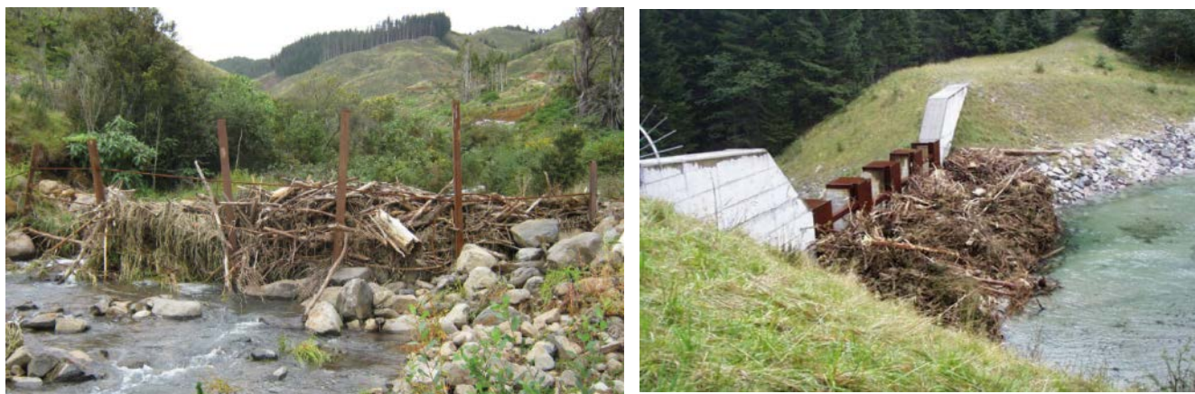
Figure 1: Left, a basic railway iron and steel rope slash trap will retain slash, with sediment building up within and behind. Right, the more permanent debris control structure will retain sediment in the pond behind, with slash being trapped at the outlet by the pillars in the structure.
