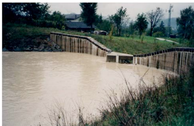
Figure 14: The photo on the left shows a retaining structure, whereby on the right looking upstream shown the sediment retained within the channel. While effective, failure to clear out the accumulated sediment has drastically changed the watercourse.
