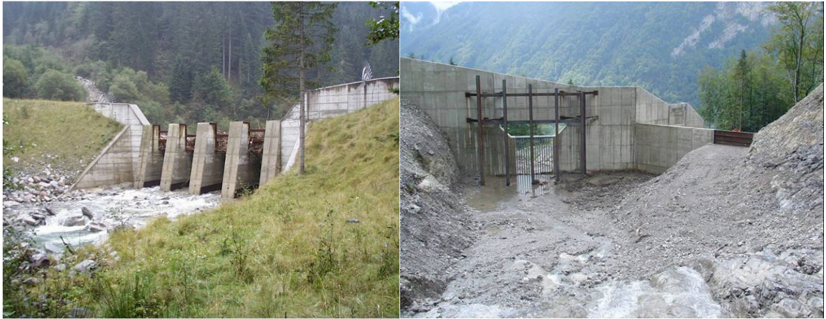
Figure 18: For this design in Italy, the calculated debris storage capacity was 12,000m 3 . The overflow weir is on the right.
