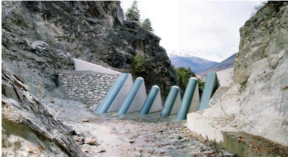
Figure 19: Front and back of a modern debris trap design. In the lower figure the sloping lead of the central design elements are clearly visible. As such larger debris elements (i.e. whole trees) will be pushed up and over in larger floods to ensure the integrity of the structure is not compromised.
