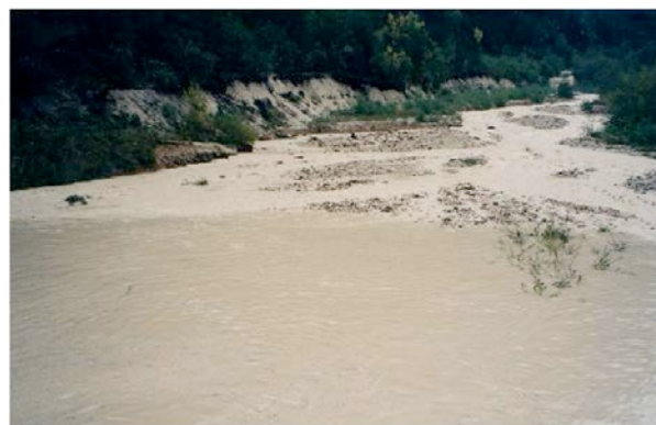
Figure 14: The photo on the left shows a retaining structure, whereby on the right looking upstream shown the sediment retained within the channel. While effective, failure to clear out the accumulated sediment has drastically changed the watercourse.
