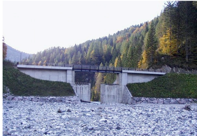
Figure 11: Debris control built into a bridge structure to avoid downstream impacts.
