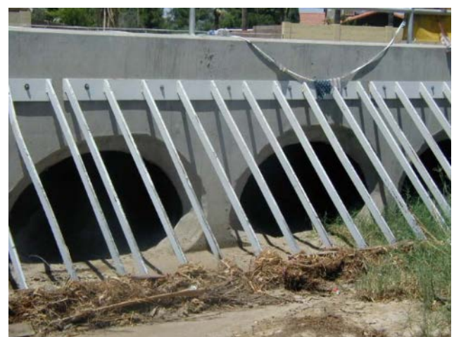
Figures 12: Two examples where a culvert is designed to primarily deflect debris, but moderate volumes of debris will also be retained.
