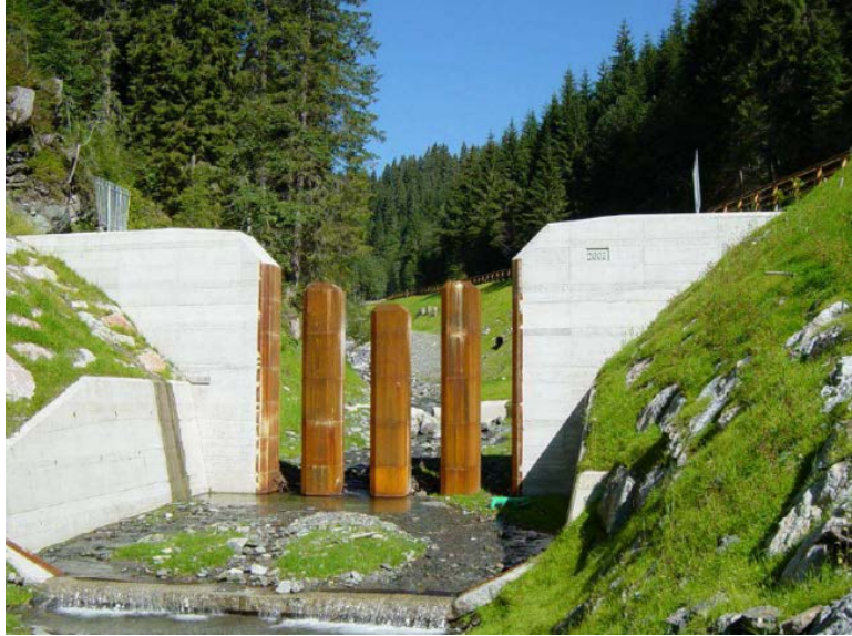
Figure 9: A debris trap design for catching a large range of woody debris with smaller apertures on the vertical columns.
