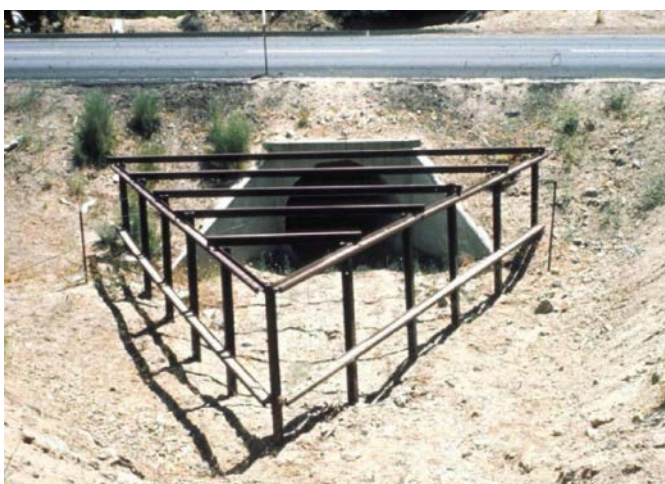
Figures 12: Two examples where a culvert is designed to primarily deflect debris, but moderate volumes of debris will also be retained.
