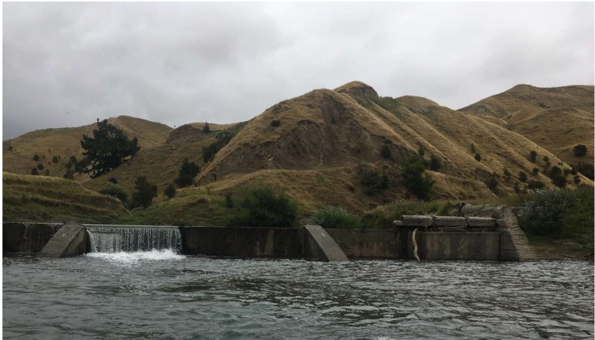
Figure 3-2: The lower weir viewed from downstream and the true left bank.
