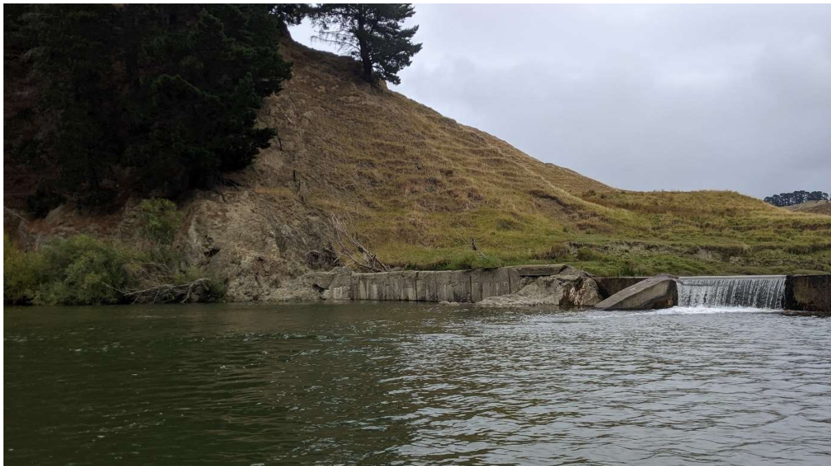
Figure 3-1: The lower weir viewed from downstream and the true right bank. Note the mudstone sill which underlies part of the weir and protrudes to the height of the weir crest in one place.
