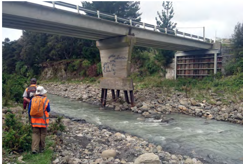
Figure 2-9 The Aorongiwai Stream (right) has experienced bed degradation (leading to undermining of bridge support), through a combination of gravel extraction and reduced sediment delivery from the upper catchment.
