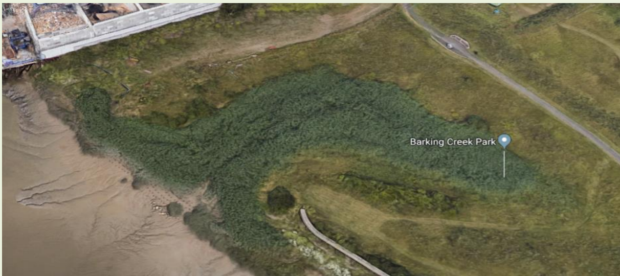
Figure 3-7: Barking Creek, Creekmouth vegetated intertidal terrace construction in 2006 (above) and Google 3D image of the results from 2018 (below). Source: https://www.estuaryedges.co.uk/case-studies/barking-creek-creekmouth/ .
