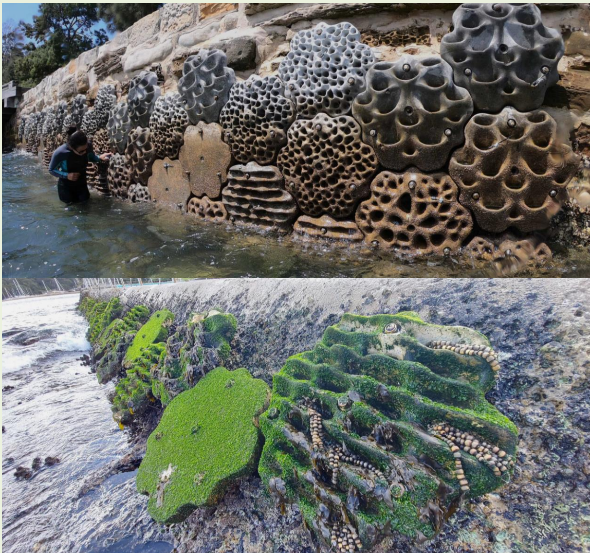
Figure 3-5: Examples of living seawalls designed in Australia and tested across three continents. Source: https://www.livingseawalls.com.au/
