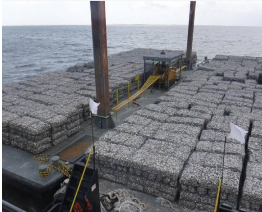
Figure 3-20: Large scale use of oyster shells in gabions. The shellfish reefs were restored near Soundview Park in the Bronx during the Billion Oyster project in New York Harbour ( https://www.billionoysterproject.org/ , Courtesy Ben Diggles, Diggsfish.com).
