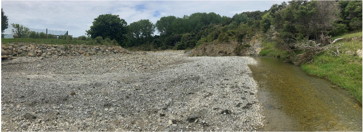
Figure 3. Finer-grained bedload, with lack of surface structuring immediately upstream of the landfill (rock revetment to the left of the image). Note protruding earthflow lobe in middle distance.
