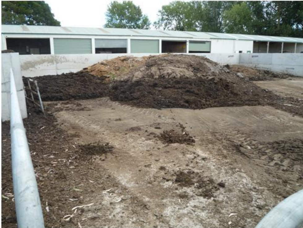
Photo 33: Solids storage bunker (photo taken months after sampling).
