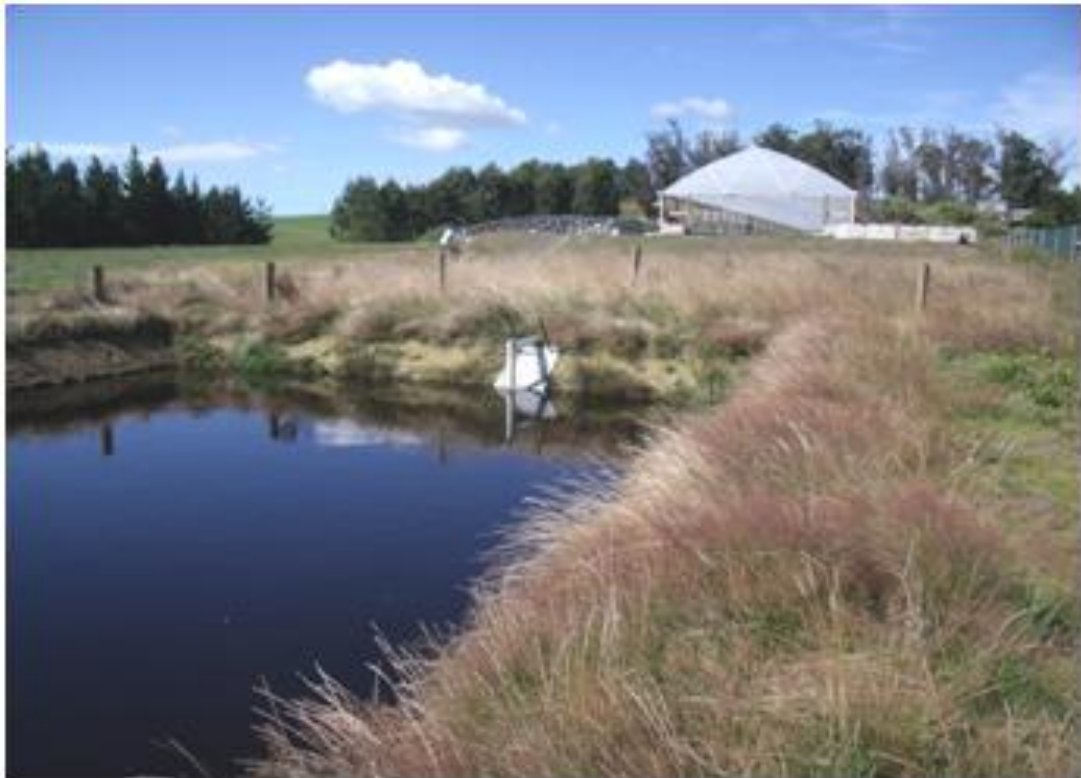
Photo 59: Pond for drained liquid from HerdHomes® Shelter.
