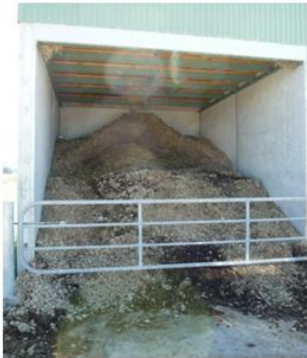
Photo 16: Covered solids bunker.
