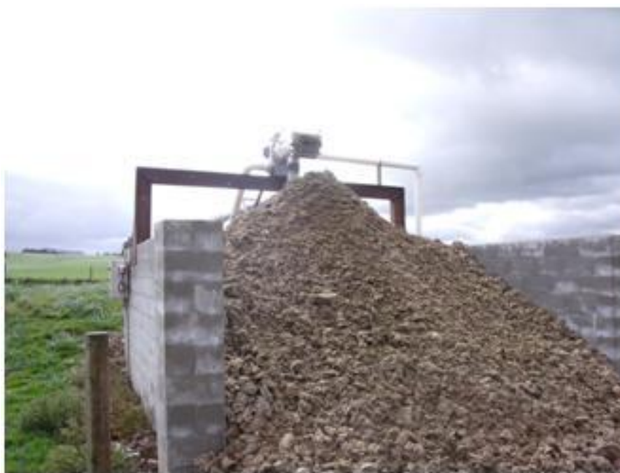
Photo 39: Mechanically separated solids in storage bunker.
