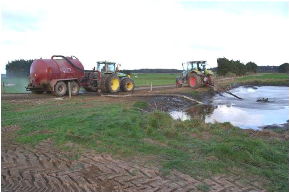
Photo 52: Weeping wall bed with liquid added. A tractor mounted stirrer (right) and slurry tanker (left) pumping out the bed with a vacuum pump
