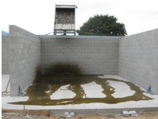
Photo 30: Static screen sited above storage bunker.
