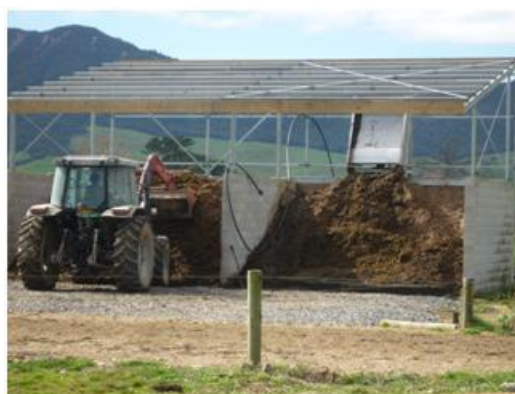
Photo 31: Screen can be moved along top of solids storage bunker. The storage bunker is in the process of becoming covered.
