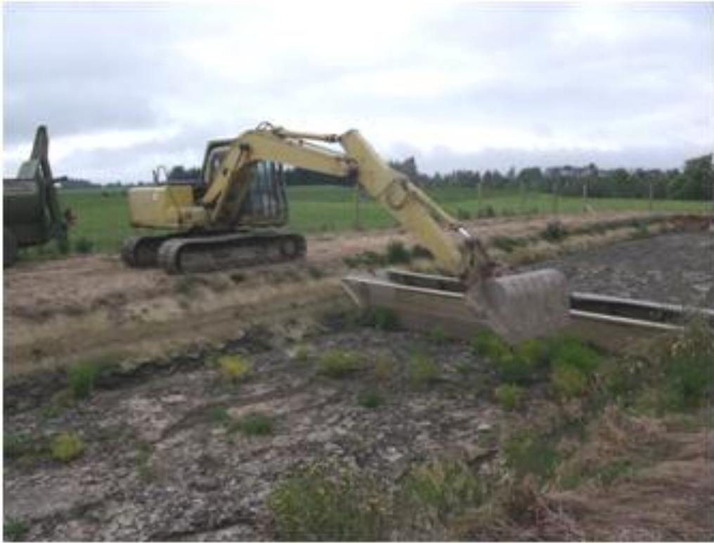
Photo 44: Excavator removing manure from the weeping wall.
