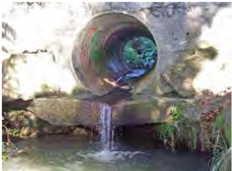
*Example of potential barriers to fish passage: perched culvert.*
