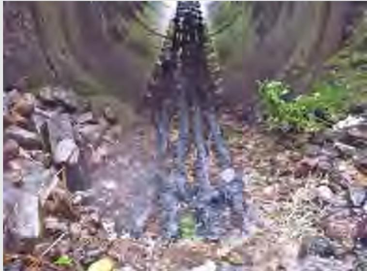
Textured ropes installed in a stream culvert to aid fish passage.
