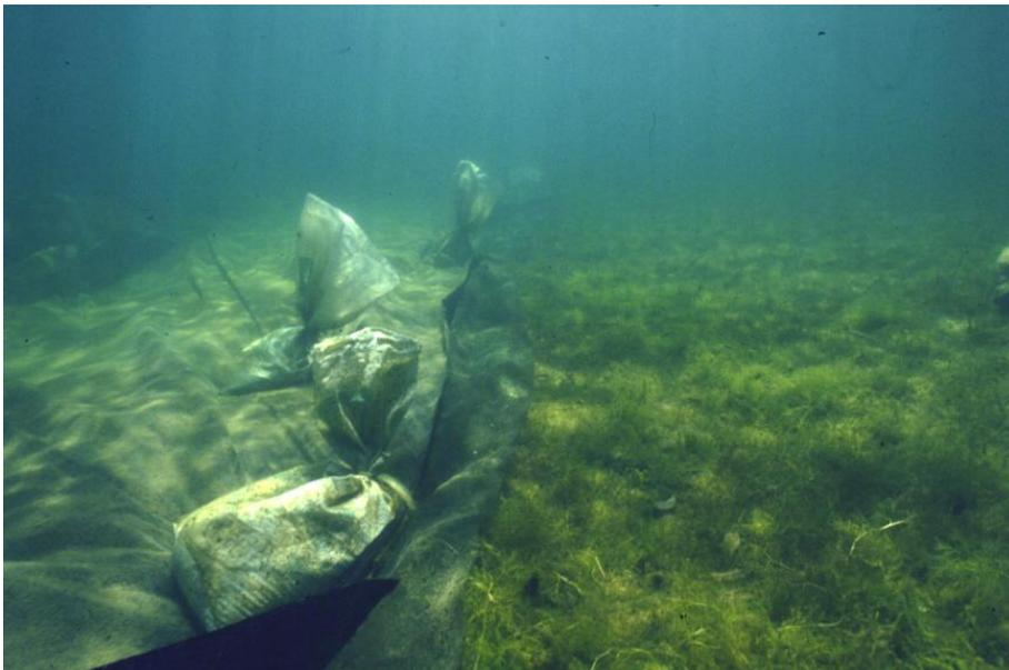
Figure 17 Placement of weed cloth held in place by sand bags (Photo: R. Wells, NIWA).
